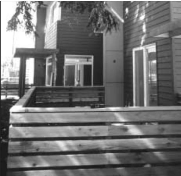
Patio built with “plastic” lumber and ACQ-treated wood.
