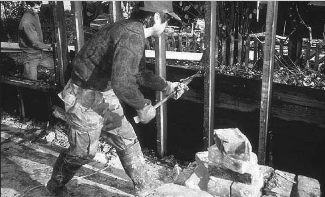
Deconstruction is an economical alternative to demolition.
