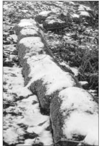
Bio-filter bags help prevent sediment from polluting waterways during construction.
